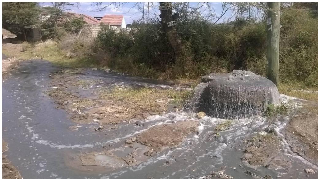
Plate 4.2: Blocked sewer manhole in Athi River spewing raw sewage into the Athi River
