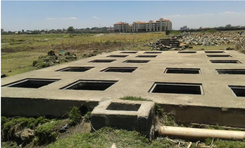
Plate 4.1: Open septic tanks (with leaking piping system) for a residential estate near the Athi River
