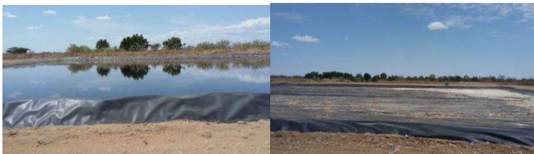
Figure 12. Evaporation ponds filled with silicate water (left), and After evaporation of the silicate water (right)
