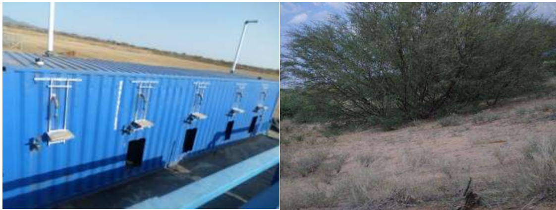
Figure 14. Effluent treatment bio-box (left) and vegetation irrigated by treated wastewater (right)
