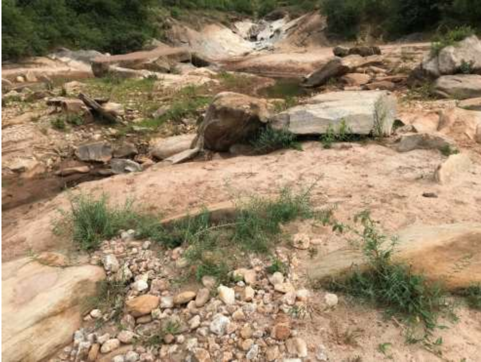
Plate 1.1: A section of the degraded Kaiti River showing traces of degraded phragmites, eroded sand and exposed rocks.
