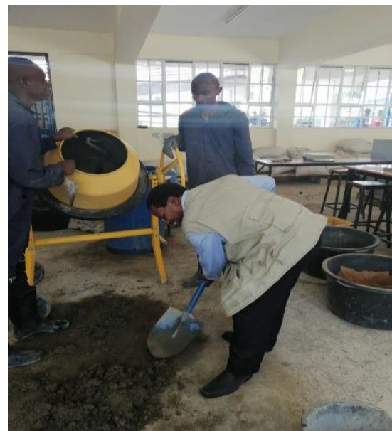
Fig 3: Hand mixing of concrete.
