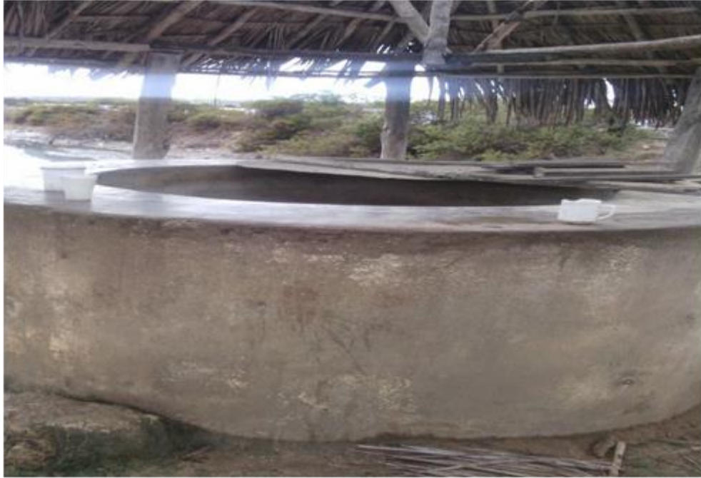
Plate 1 An open well in Gongoni area of Kilifi County (photograph taken by author)
