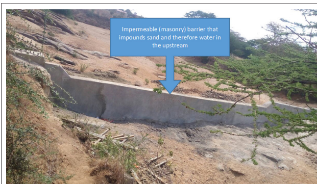
FIGURE 4 | A newly built sand-storage dam.
