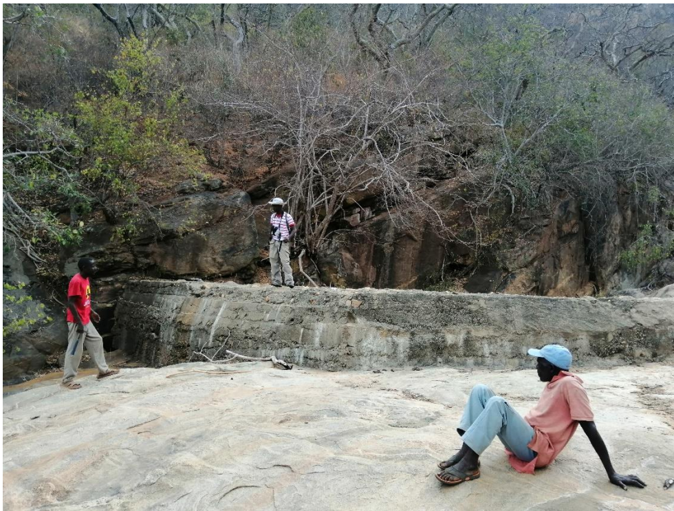
Plate 4. 36: A dam constructed on a migmatite floor to collect rainwater
