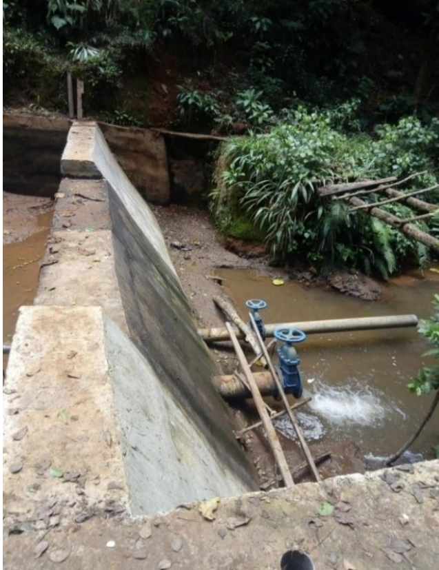
Plate 4.2: Weir constructed across Kimakia River Ririndia
