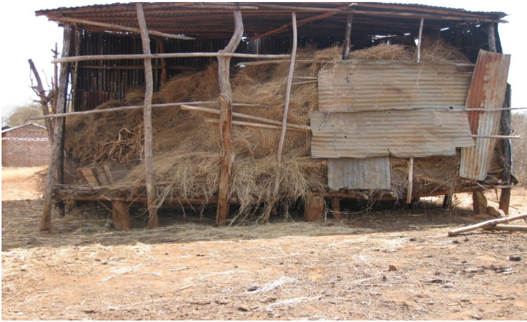
Figure 4.13: Adopted Hay Barn used for storage of feedstuffs
