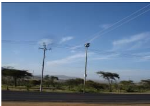
Plate 3.2: Street lights outside the Alim High School gate.
