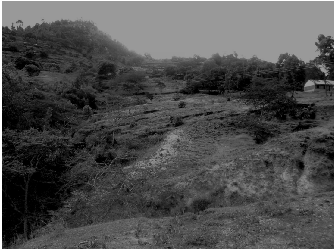
Plate 4.4: Gully formation from soil and water erosion emanating from road infrastructure in Nunguni
