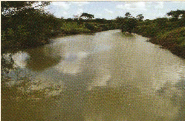
Water dam Constructed through public private partnership project.
