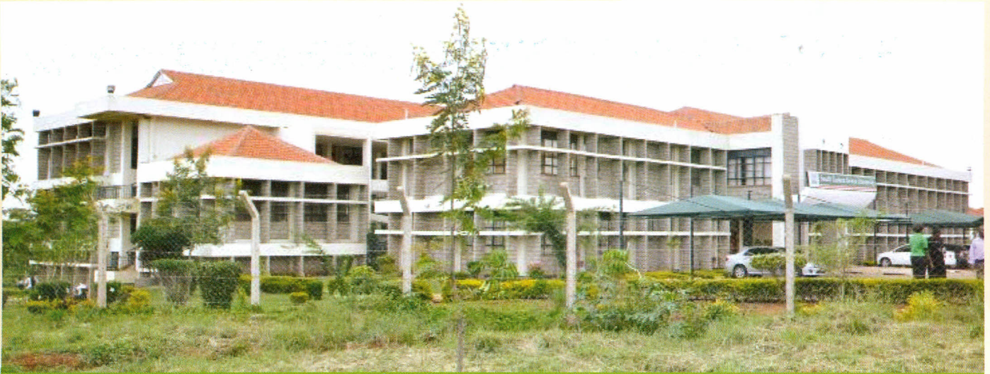
Tuition and office block I
