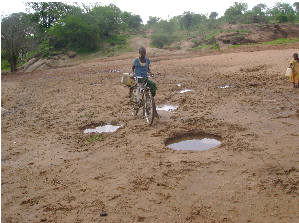
Plate 2: Water abstraction from a sand dam constructed elsewhere in Kitui District.
