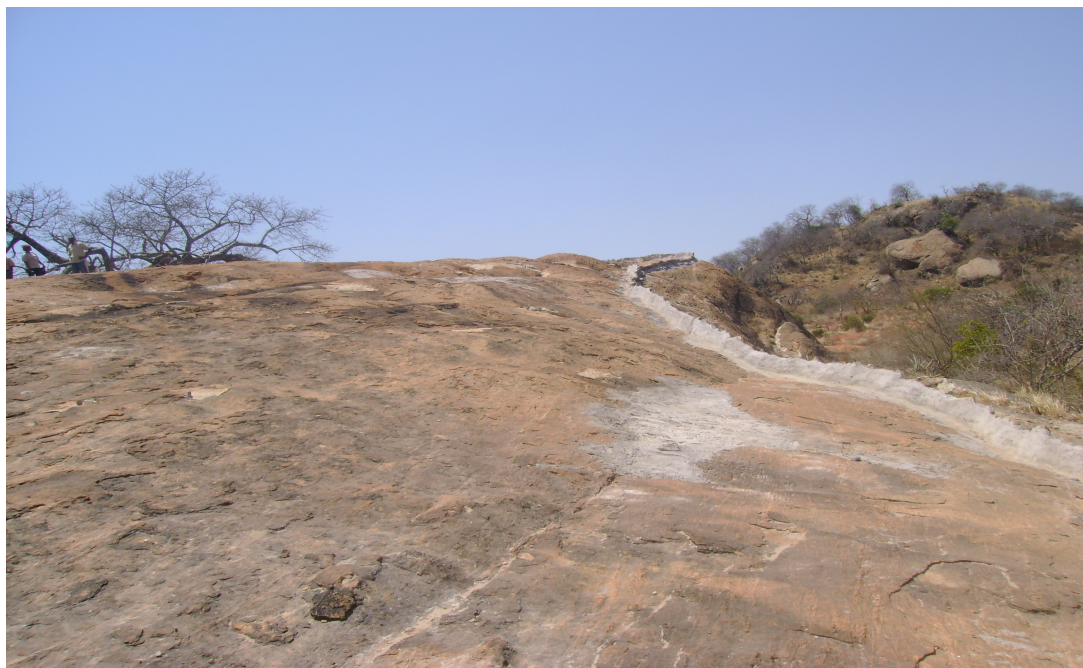
Plate 3: A typical rock catchment constructed elsewhere in Kitui District.
